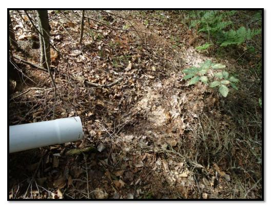
Figure 5: Release of wastewater directly on to property with no septic system
